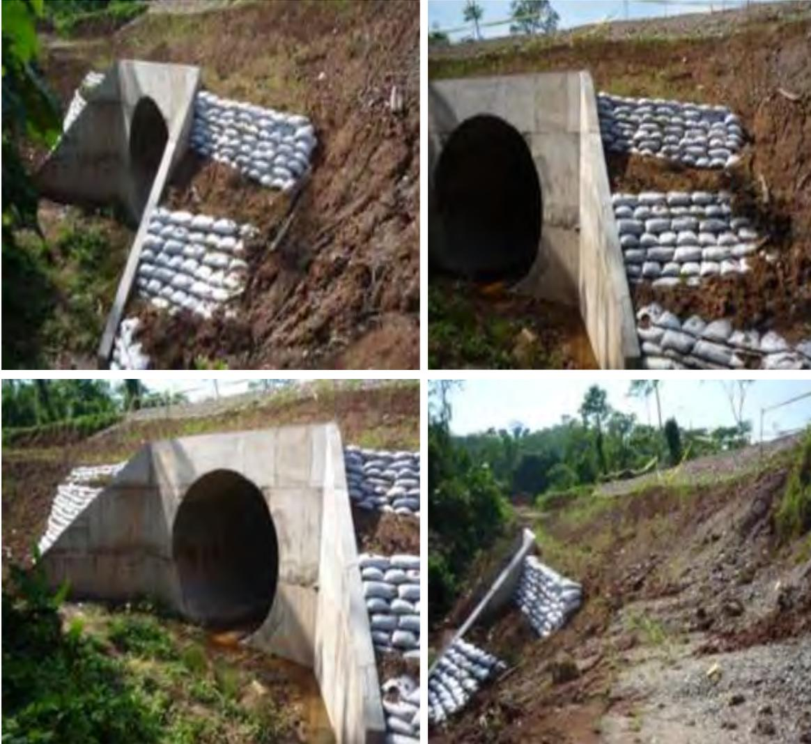
**Fig.3.21 : Alcantarilla terminada**
