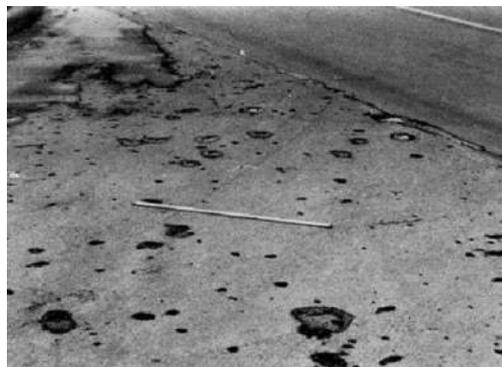
**Figura 20.** Popouts. *Fuente: ASTM D6433-03.*
