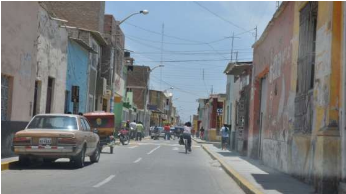
Figure 3, Intersection in Chiclayo, car, mototaxi, motorcycle, bicycle, wheelbarrow and pedestrians. Speed bump prior to intersection and illegal ramp.
